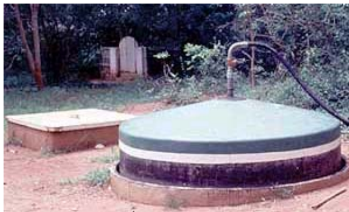
Fig. 1 Fixed Dome Type Bio-Gas Plant
