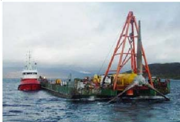
Fig 5 : Hammerfest Strøm horizontal-axis turbine about to be deployed in demonstration project, Northern Norway, 2003.
